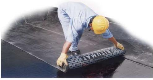
BITUMAT APP Modified bitumen rolls shall be stored vertically on ends, on a flat surface, one high without super positioning, in a dry ventilated room. Rolls shall not be laid flat until ready for installation.
